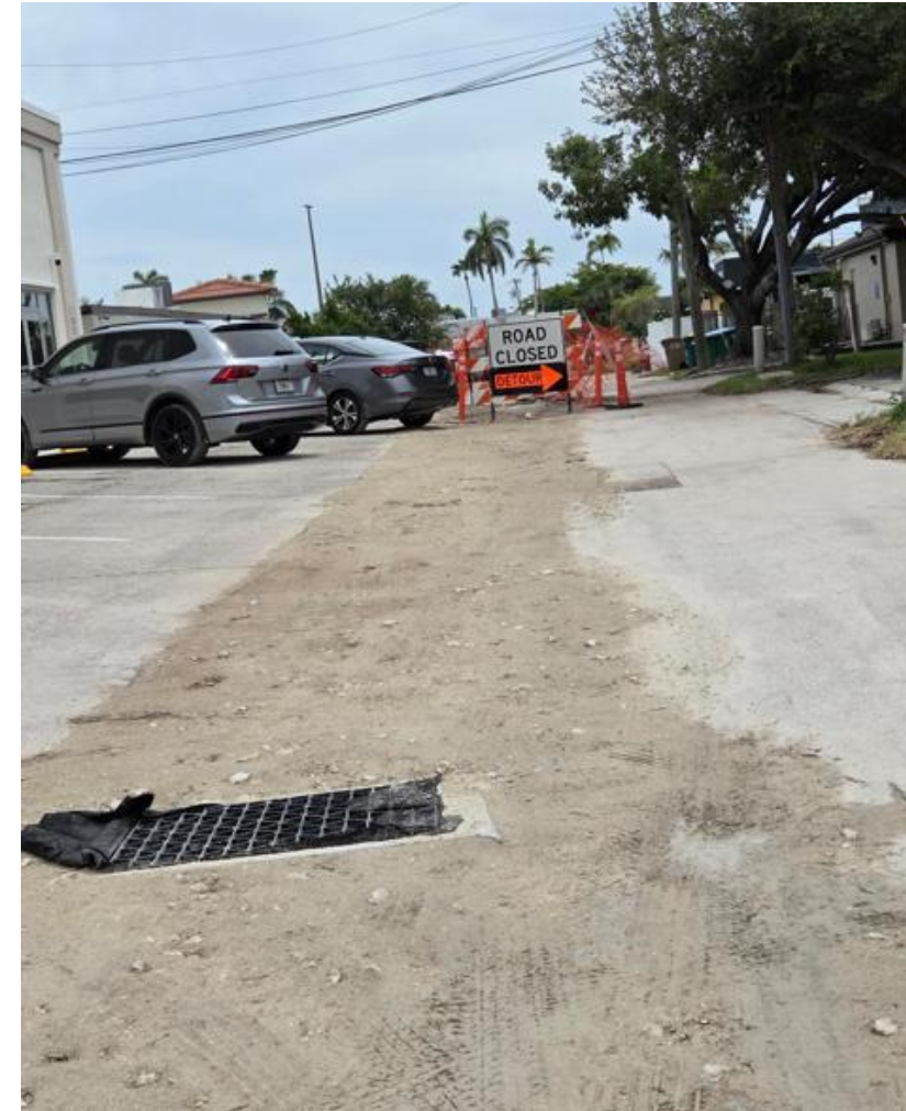
Alley #360 - Under Construction
